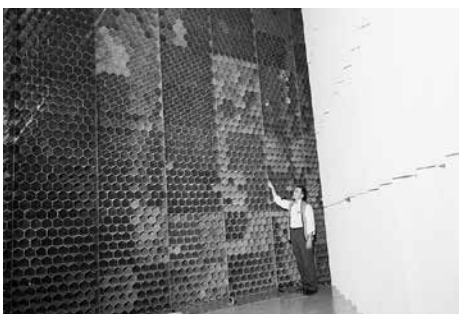
This honeycomb installation is from a Boeing transonic wind tunnel in the 1960s. © Boeing. All Rights Reserved.
